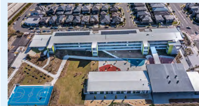
Aerial view of Edmondson Park Public School
