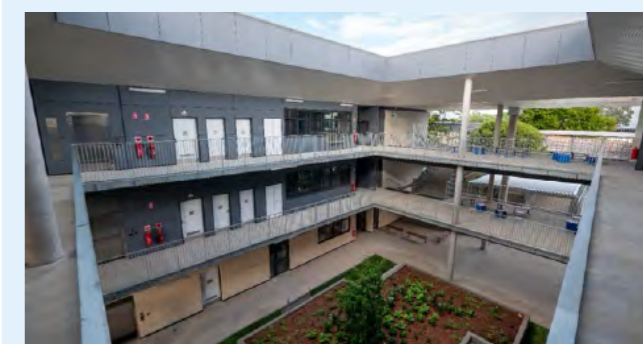
Pendle Hill High School upgrade
