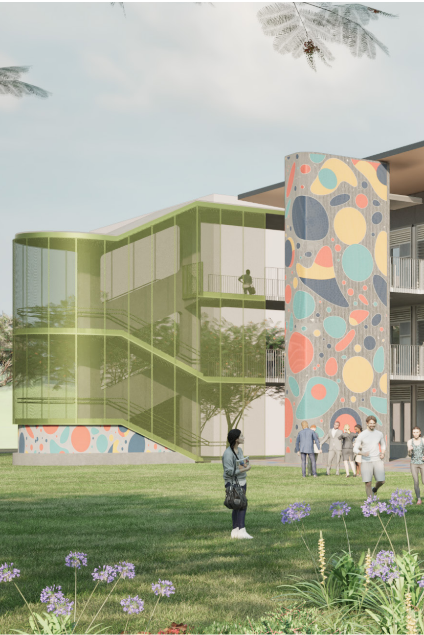
Concrete painted with artwork
