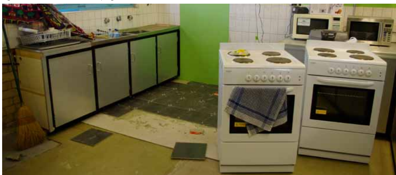
Figure 3.7 Kitchen construction in progress
